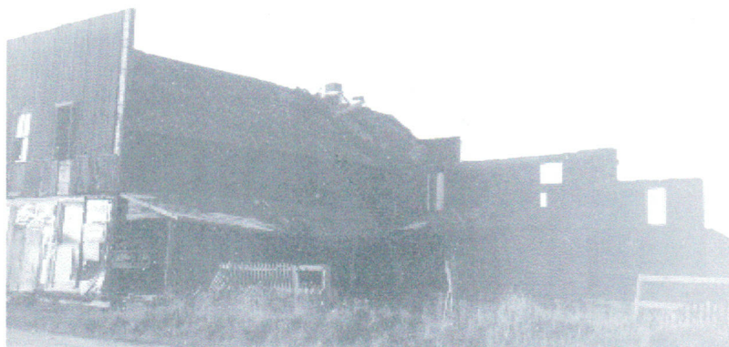
Pic 38: Demolition of General Store and Bates home
