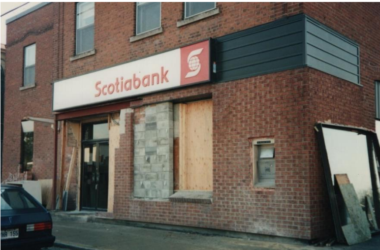
Pic 14: Installation of ABM, 1995
